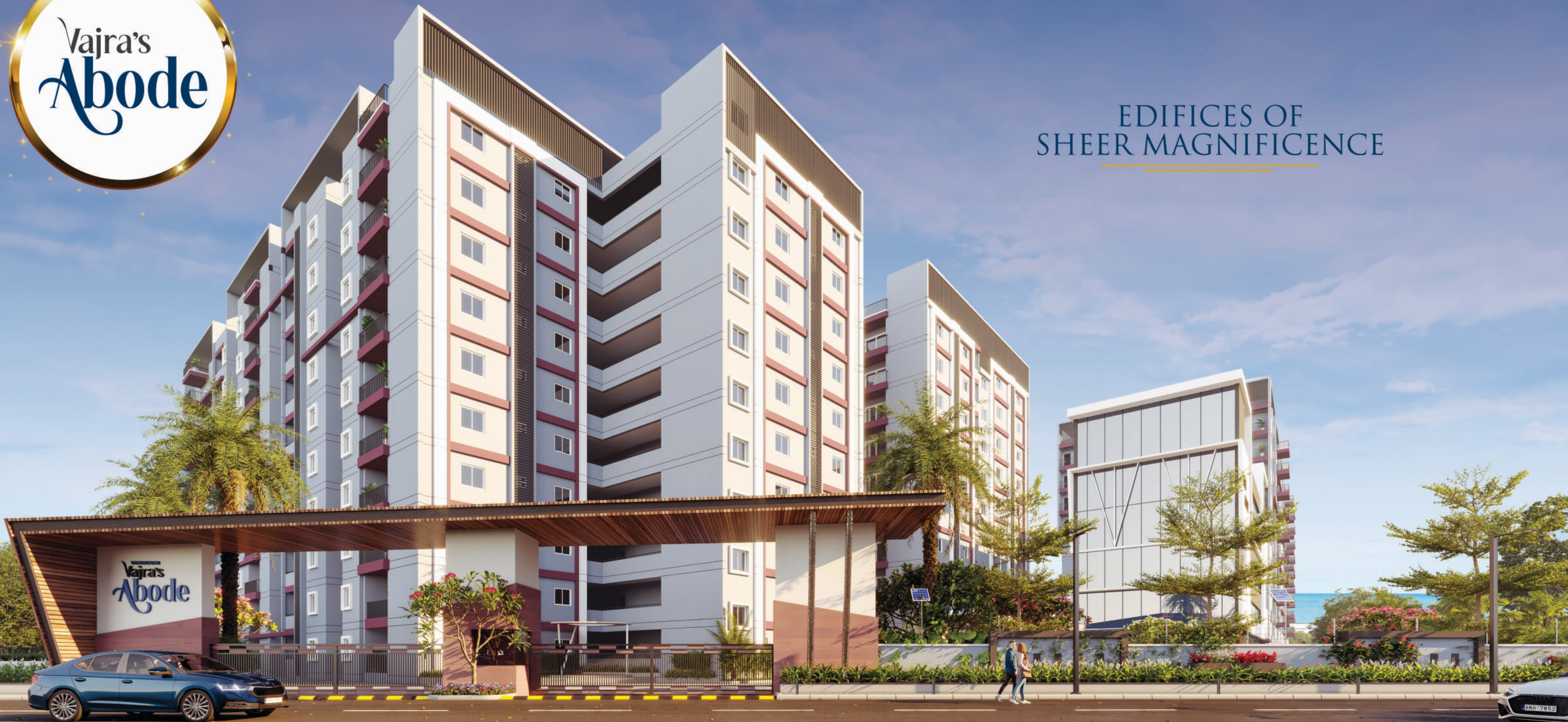
Entrance Podium to Block - B, C & D
